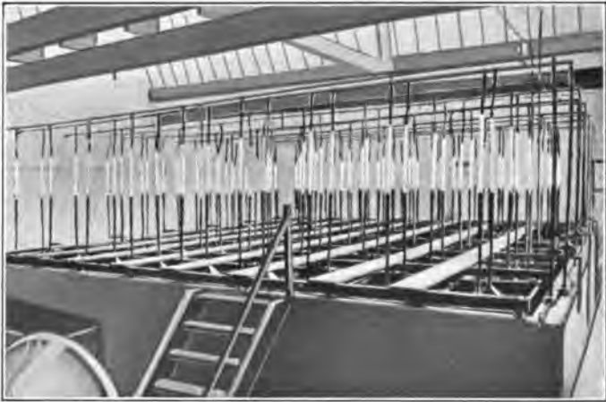
FIG. 109. Battery of Garuti generators.
